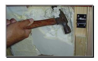
It is important to have clear access to the crack area from the backside of the spa. You will have to remove the following parts:
